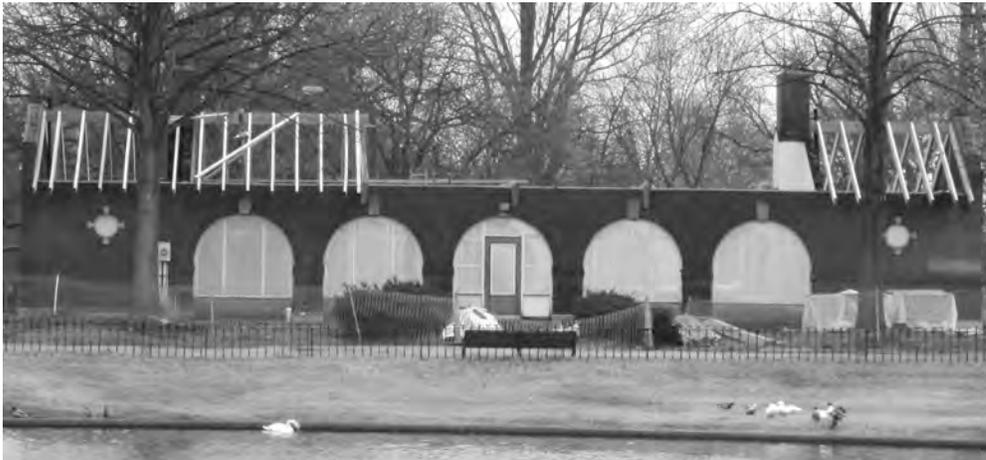
*New rafters going up have eave ends cut to match the original blueprint design.*
