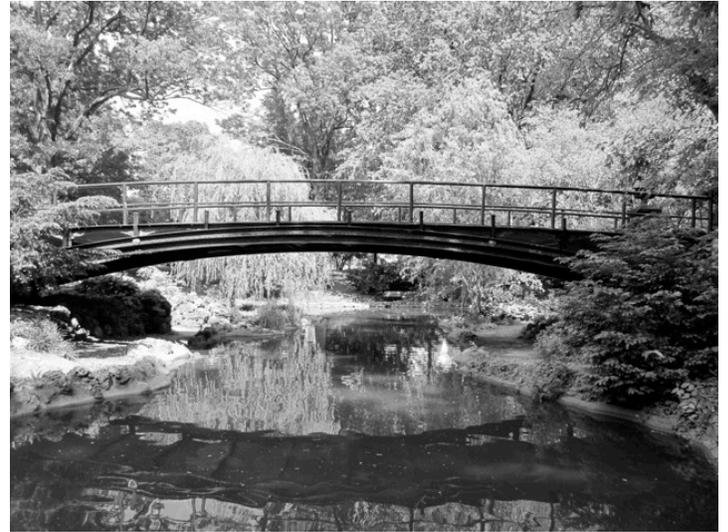
Engineering inspection showed the steel supports and expansion joints were either missing or rusted through. The main arches over the lagoon were a major concern and needed to be reinforced. New arches were made by bending 6 inch I-beams to match the curve of the old arches. These arches were welded under the existing arches to support the decking of the bridge. New footings with embedded bolts for attachment plates were poured to support the arches.
