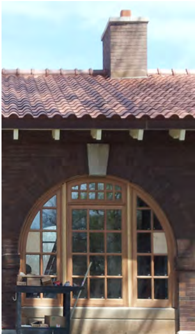
New windows as seen from the exterior.
