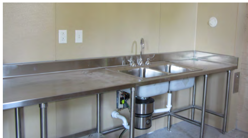
The partially finished catering kitchen sink area in the Boathouse.
